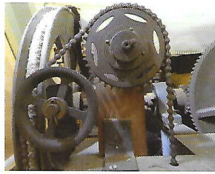
Investigating Alford Manor House lift
