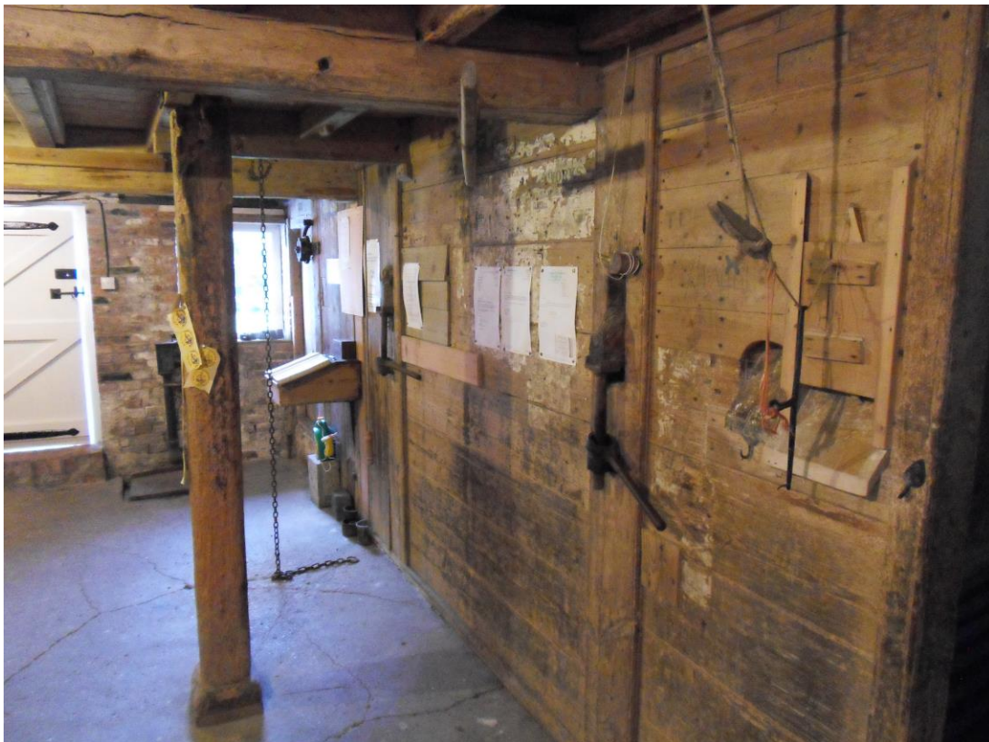
Fig.9 The ground floor depicting the boarded gear box with meal spouts & millstone gap adjusting screws; note the mill box desk with the ratchet & pawl above to operate the waterwheel gate mechanism.
